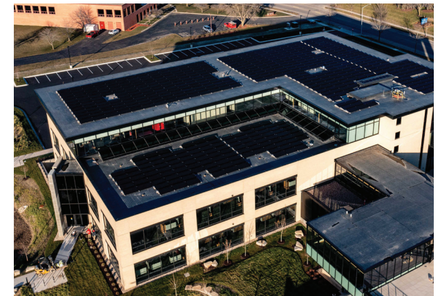
Aerial view of UW Credit Union's new administrative campus in Madison, exhibiting the 560+ rooftop solar panels placed to reduce greenhouse gas emissions. Photo courtesy of Findorff.
